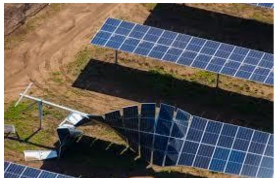
Damaged solar panels at Oakey solar plant after strong winds. Image via -magazine-australia.com
