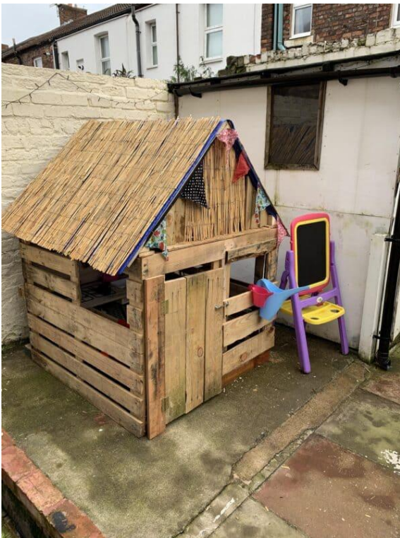
Figure 7 (left) – Kids Pallet Playhouse, built using four pallets
